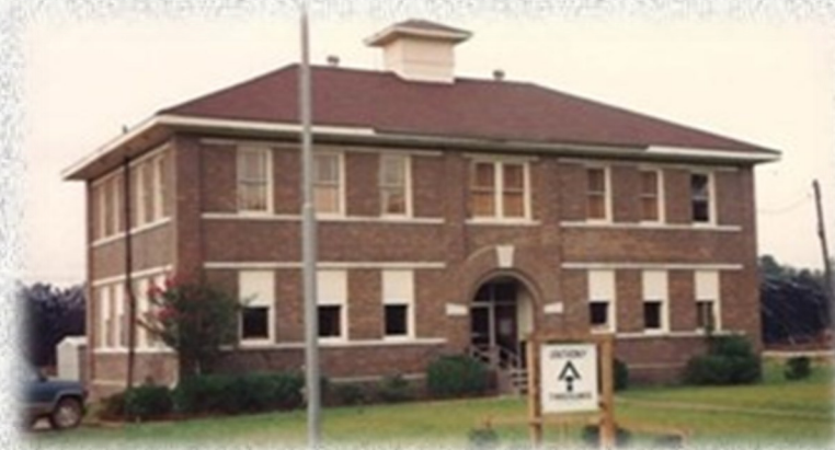
Anthony Timberlands office in the Beirne school building
